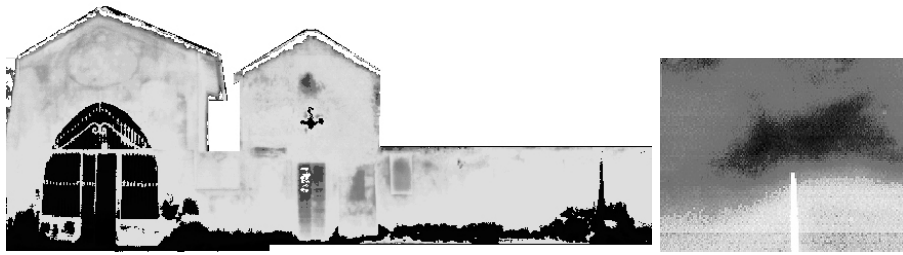
Fig. 1. Moisture detection in outdoor and indoor condition.
