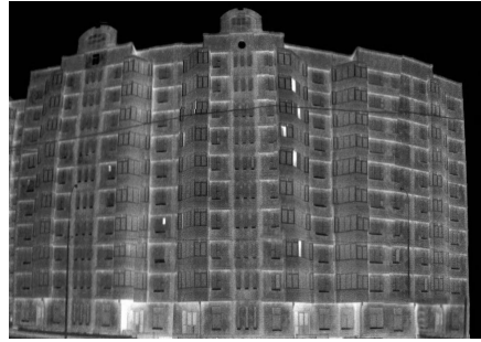
Fig.4. A typical thermogram of outdoor guarding construction of a building.
