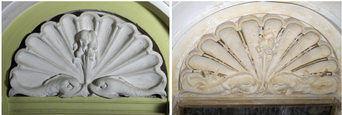
Fig. 5. Stuccowork in Ciechocinek (Poland). On the left side picture a fragment covered with white wash, on the right side – gilding uncovered after cleaning
