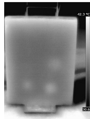
Fig. 7. Infrared picture of the slab : passive thermography (the only source of heating is the sun)
