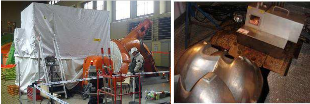
Figure 9: prototype PTC under laser protection tarp during Pelton wheel inspection at Passy
