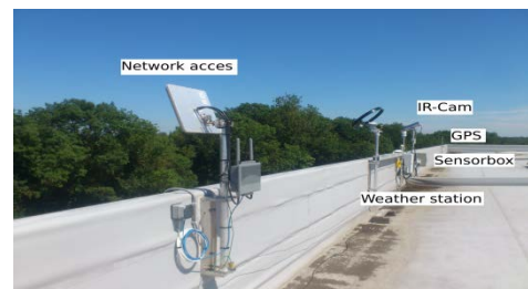
Fig. 6 Schematic view of the system and the roof layout
